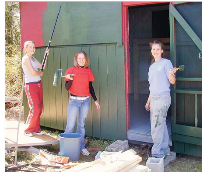
Ewell-St. Paul's gets a new coat of paint
